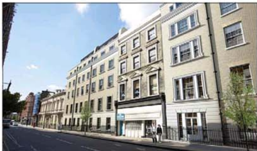
Benchmark: by October, One Housing Group will have turned former Marylebone magistrates' court into 60 new apartments for rent and shared ownership
