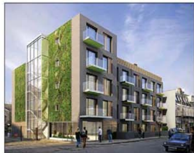
Keep it local: 32 affordable flats for local workers are being built by Pocket in Fermoy Road, W9. Visit pocketliving.com
