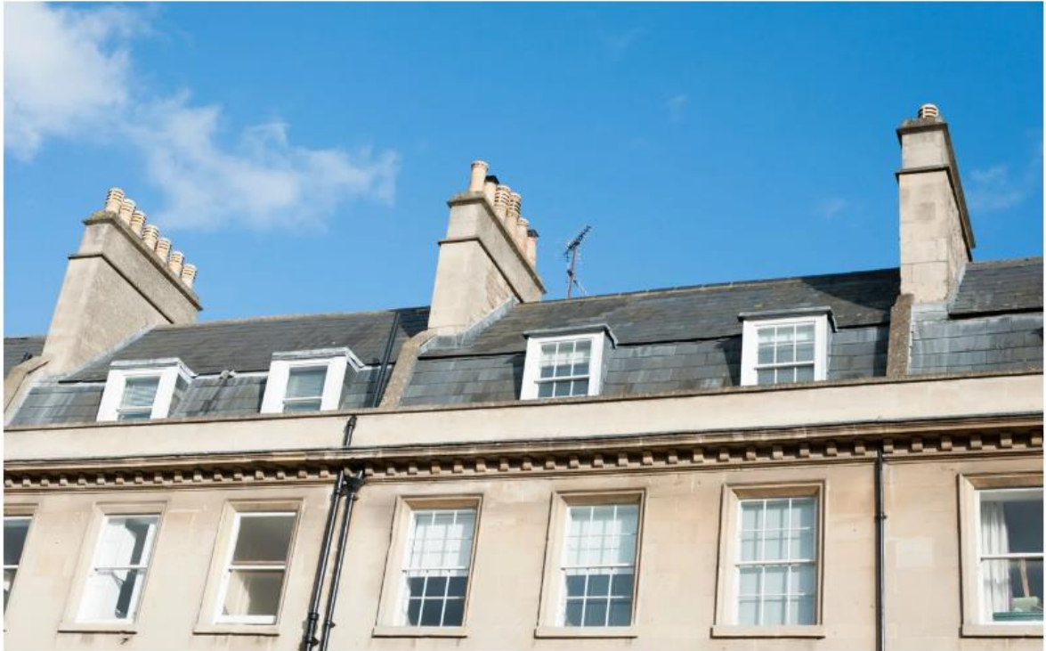
The government wants to encourage mansard roof extensions
